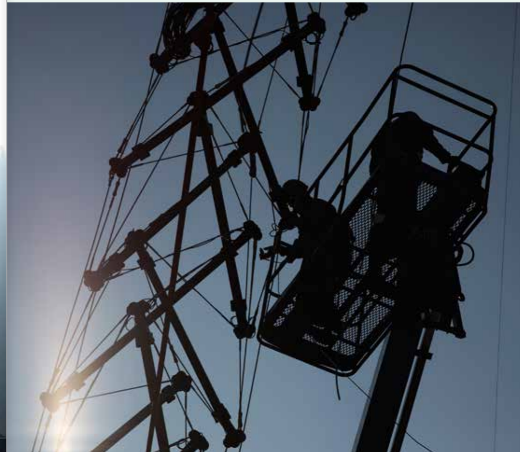
↑ Inox-Litze Toron Inox Stainless steel strand 1 x 19 E = 1,4 - 1,7 · 10 5 N/mm 2
