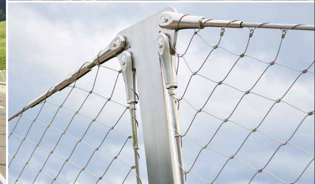
Hundwilertobelbrücke, Appenzell AR (CH)
